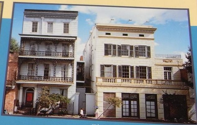
The same two buildings, 1993
